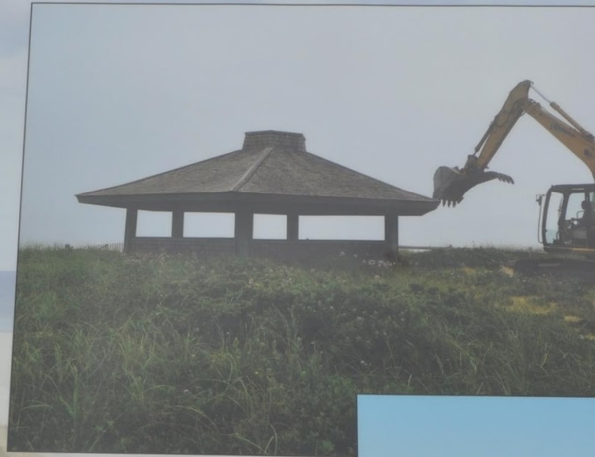
Demolition of the exhibit shelter, July 2013
